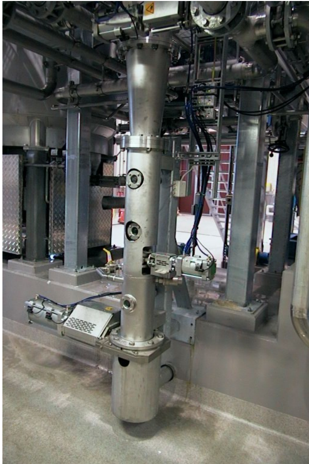
Installation i RTC Pilot Plant
